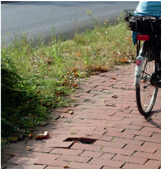
Cycle track with structural shortcomings – Kurfürstenallee
