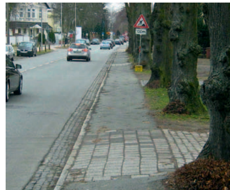
Poor condition of the cycle track in Huchtinger Heerstraße
