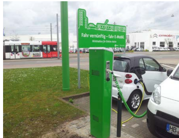
Abb.6: Move About Station (BSAG Zentrum)
